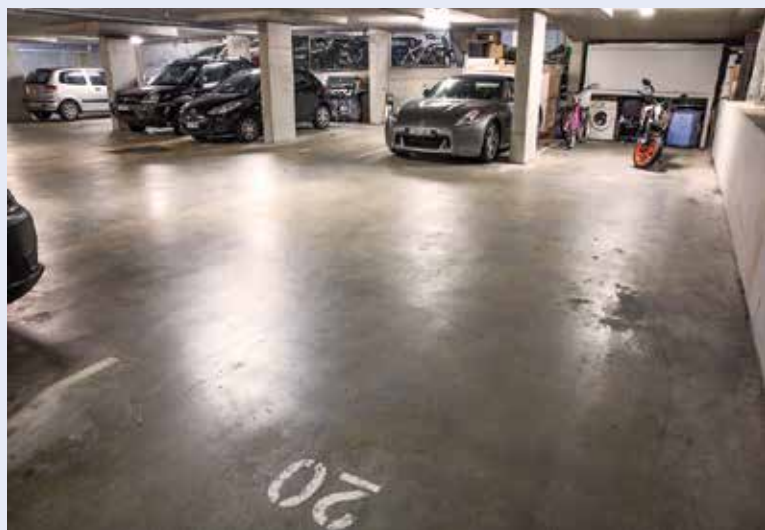
Bãi đậu xe Pittwater Road Residential Manly, Úc
